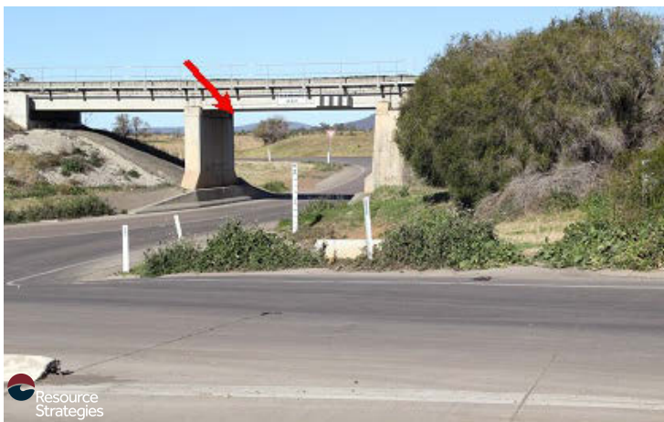
PLATE 6: Recommendation 6 West Along Quia Road to Railway Underpass Obstruction marker missing over westbound travel lane – not required by Standard, but one provided over eastbound travel lane.
