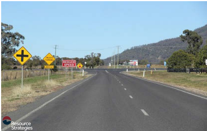
PLATE 3a: Recommendation 3 Approaching Oxley Highway on Blackjack Road Incorrect use of sign warning of four way intersection on the minor road, and one additional sign obscured by the "Reduce Speed" guide sign.
