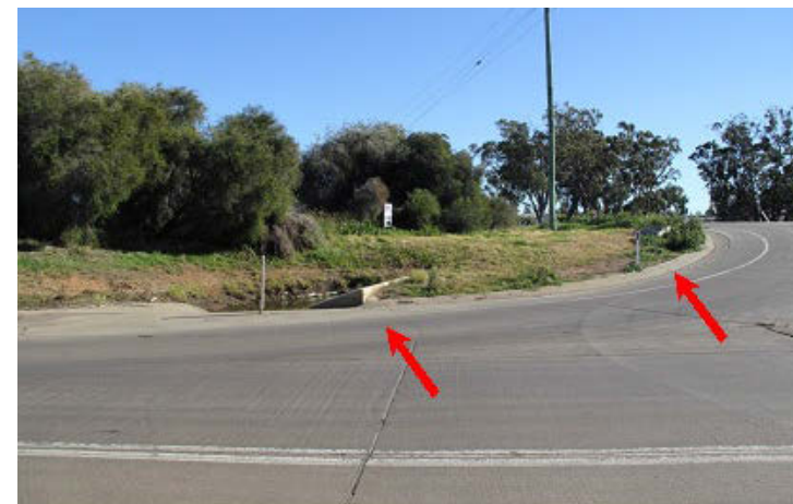
PLATE 7: Recommendation 7 Intersection of Quia Road and Torrens Road Note two unprotected culvert headwalls close to the edge of the carriageway.
