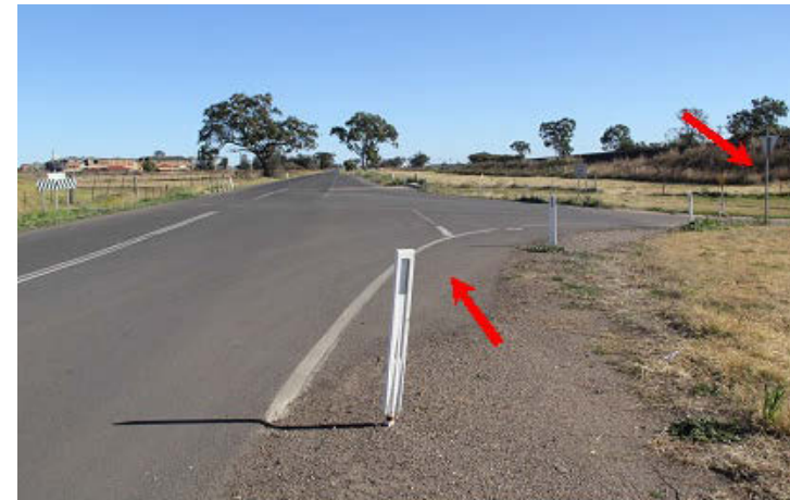
PLATE 5: Recommendation 5 Along Quia Road from East of Farrar Road (Ross Road) Intersection Conflicting non-standard "stop" line and "give way" sign on Quia Road.
