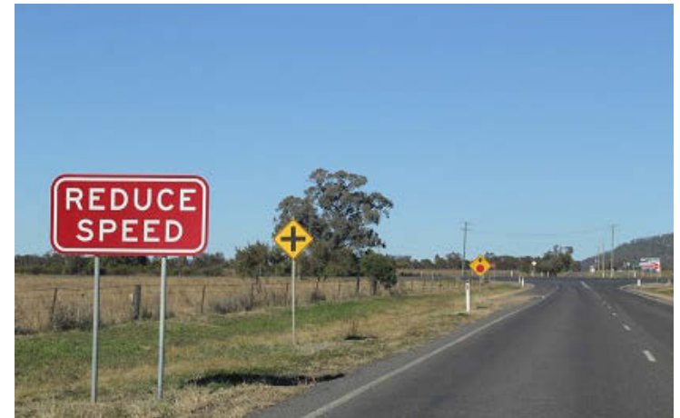
PLATE 3b: Recommendation 3 Approaching Oxley Highway on Blackjack Road Incorrect use of sign warning of approaching four way intersection on the minor road, and sign obscured on approach.
