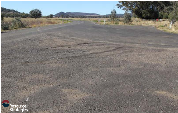
PLATE A3: Recommendation E Intersection of Coocooboona Lane and Sunnyside Access Looking East Poor road surface and non-standard line marking. Double centre lines on Coocooboona Lane through the intersection have been removed but remain visible.
