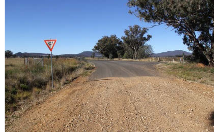
PLATE A2: Recommendation B Approaching Sunnyside Access Intersection from Coocooboona Lane Southbound Give way sign approximately 25-30m in advance of intersection and no visible give way line for traffic approaching from Coocooboona Lane southbound.
