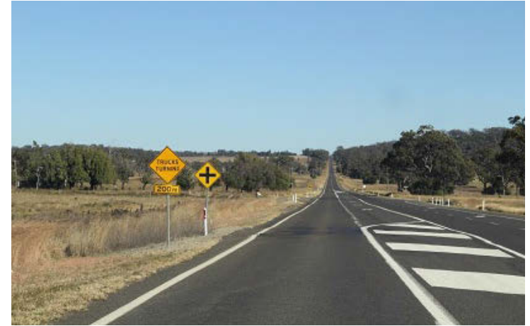
PLATE 2: Recommendation 2 Approaching Coochooboonah Lane on Oxley Highway from Gunnedah Note use of superseded "TRUCKS TURNING" sign.
