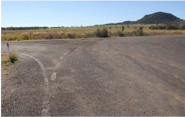
PLATE A1: Recommendation A Exiting from Sunnyside onto Coocooboona Lane Poor road surface and non-standard line marking in poor condition.
