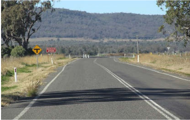
PLATE 1: Recommendation 1 Approaching Oxley Highway Intersection on Coochooboonah Lane Incorrect use of warning sign for approaching tee intersection at a four way intersection.
